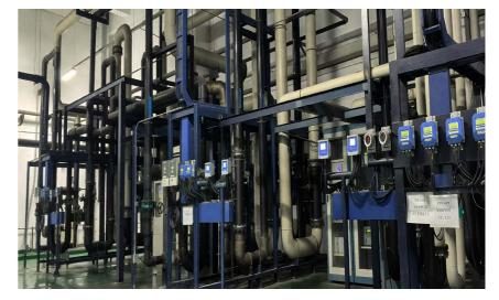
Reclaimed water replacing tap water for ultrapure water production at the BOE Beijing Gen 8.5 TFT-LCD production line
